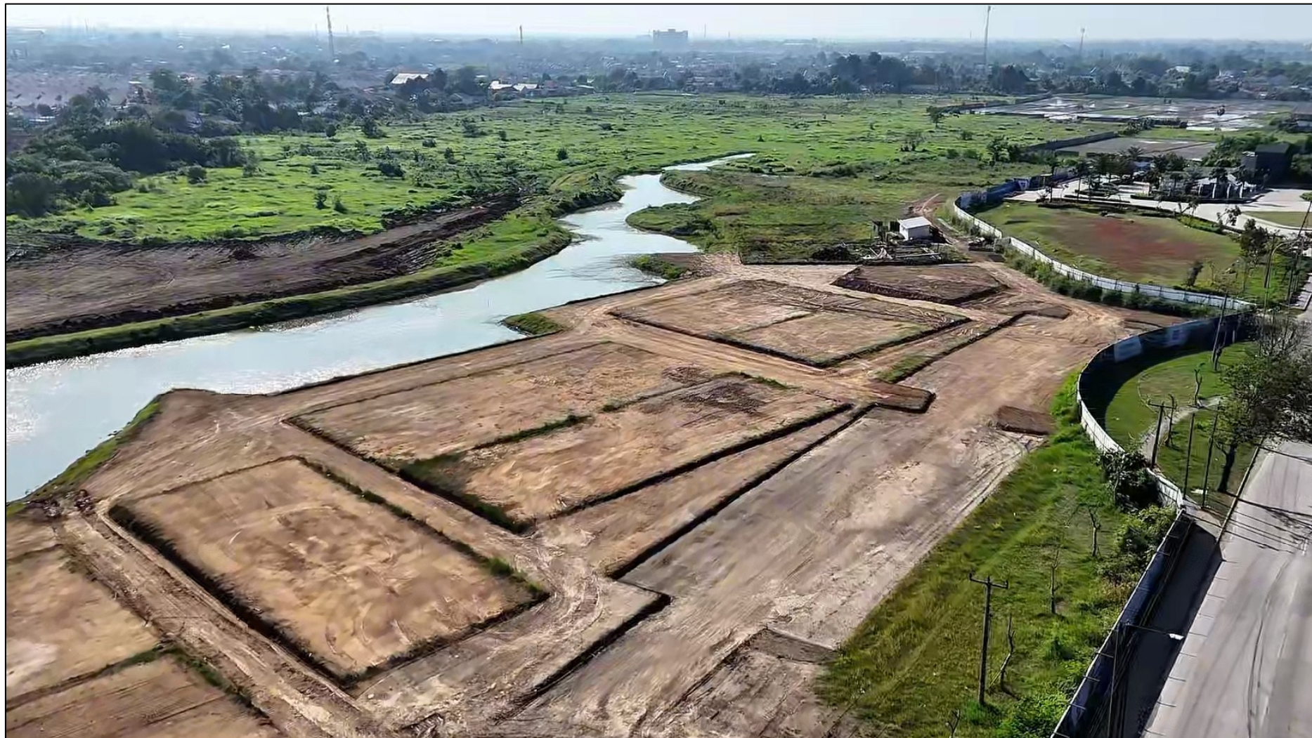
Commercial Shophouse Area - Land Cutting Progress
