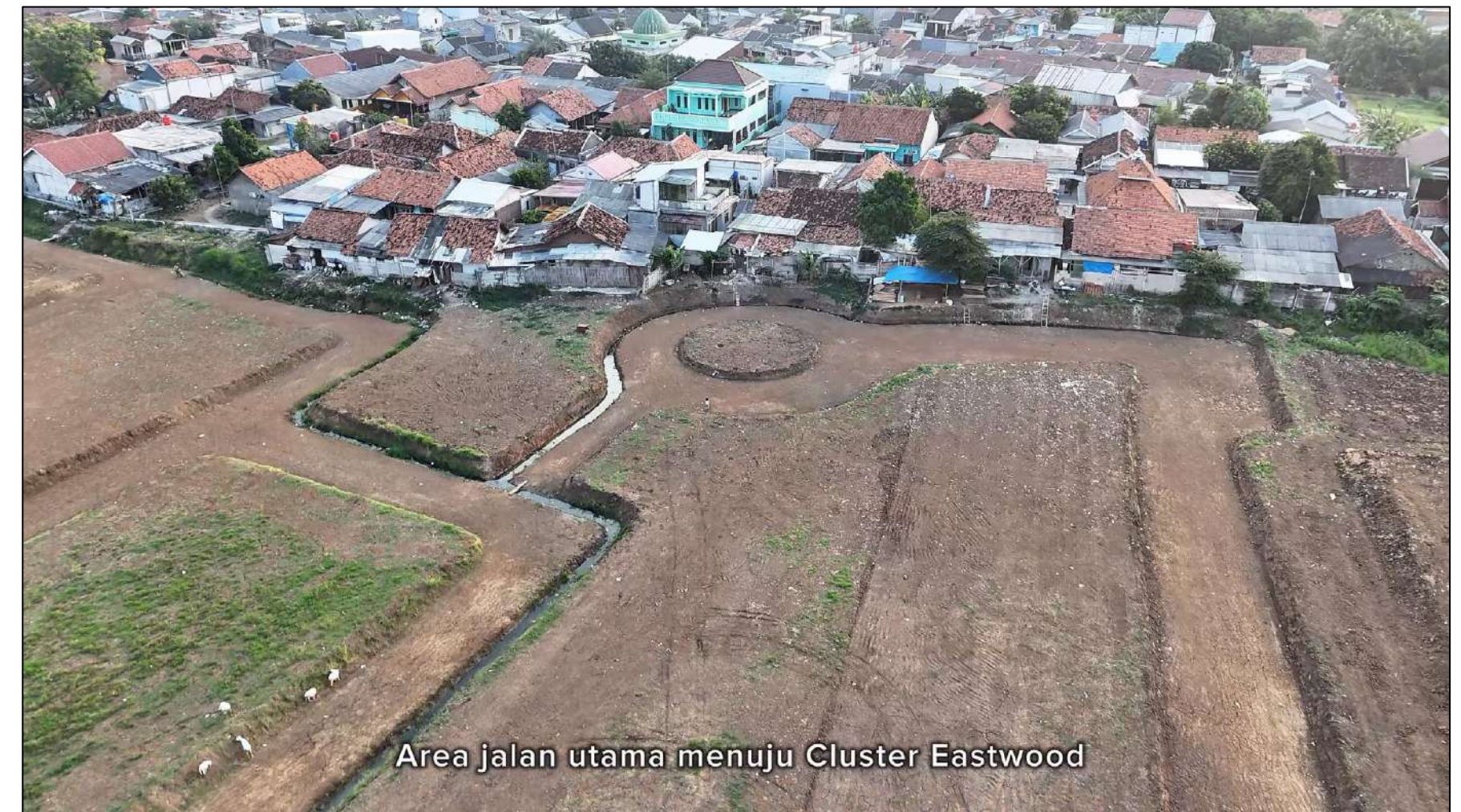
Eastwood Cluster - Road Formation Progress
