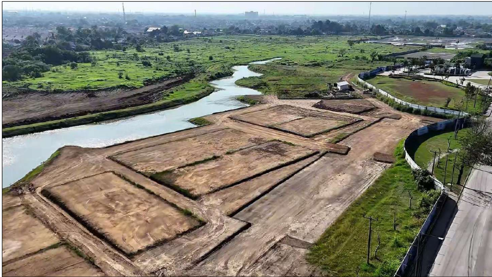
Commercial Shophouse Area - Land Cutting Progress
