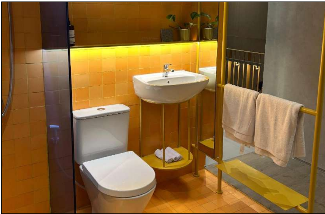
Interior Finishing for the Bathroom Area
