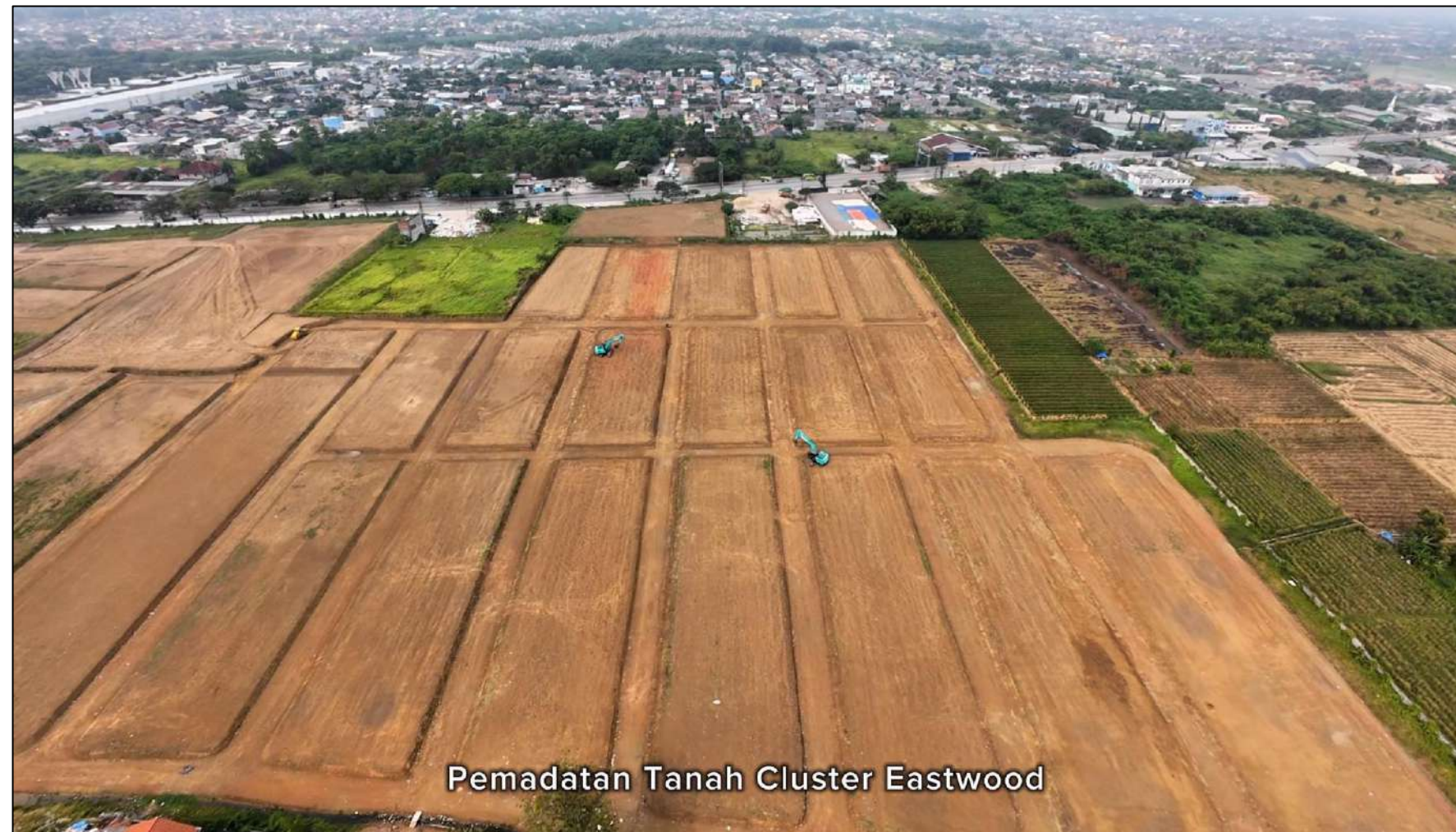
Eastwood Cluster - Land Cutting Progress
