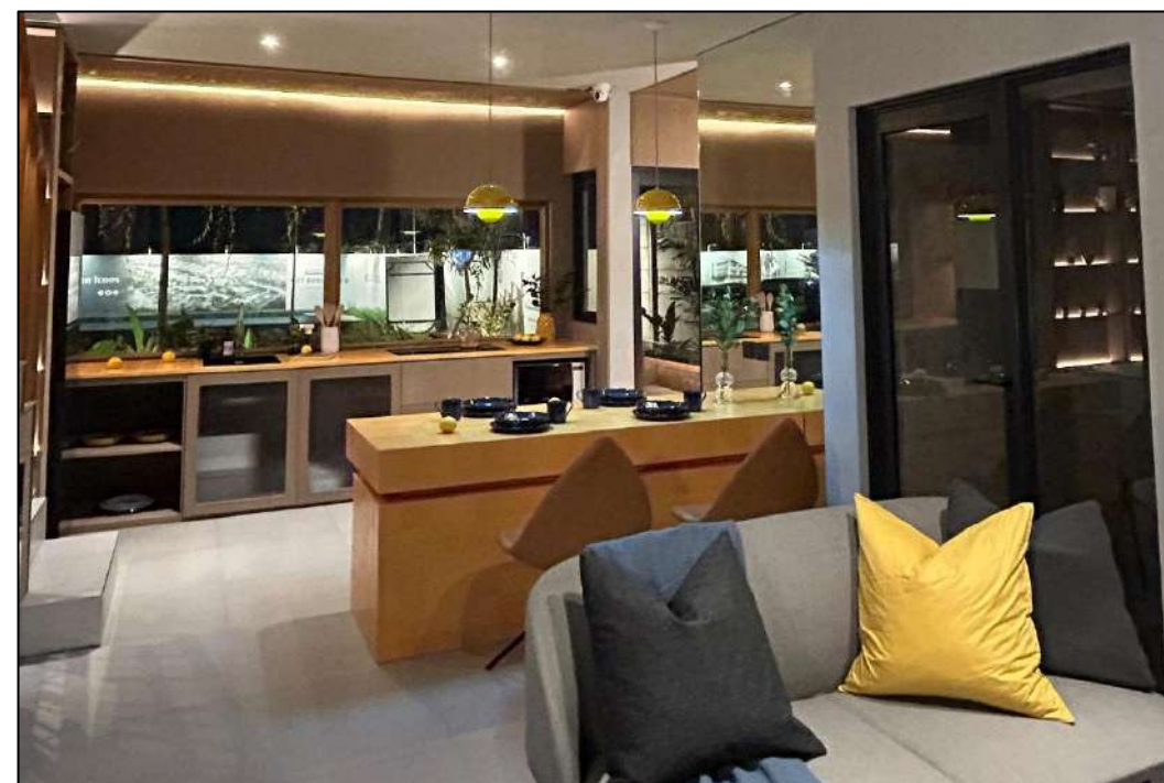
Living Room Interior Finishing
