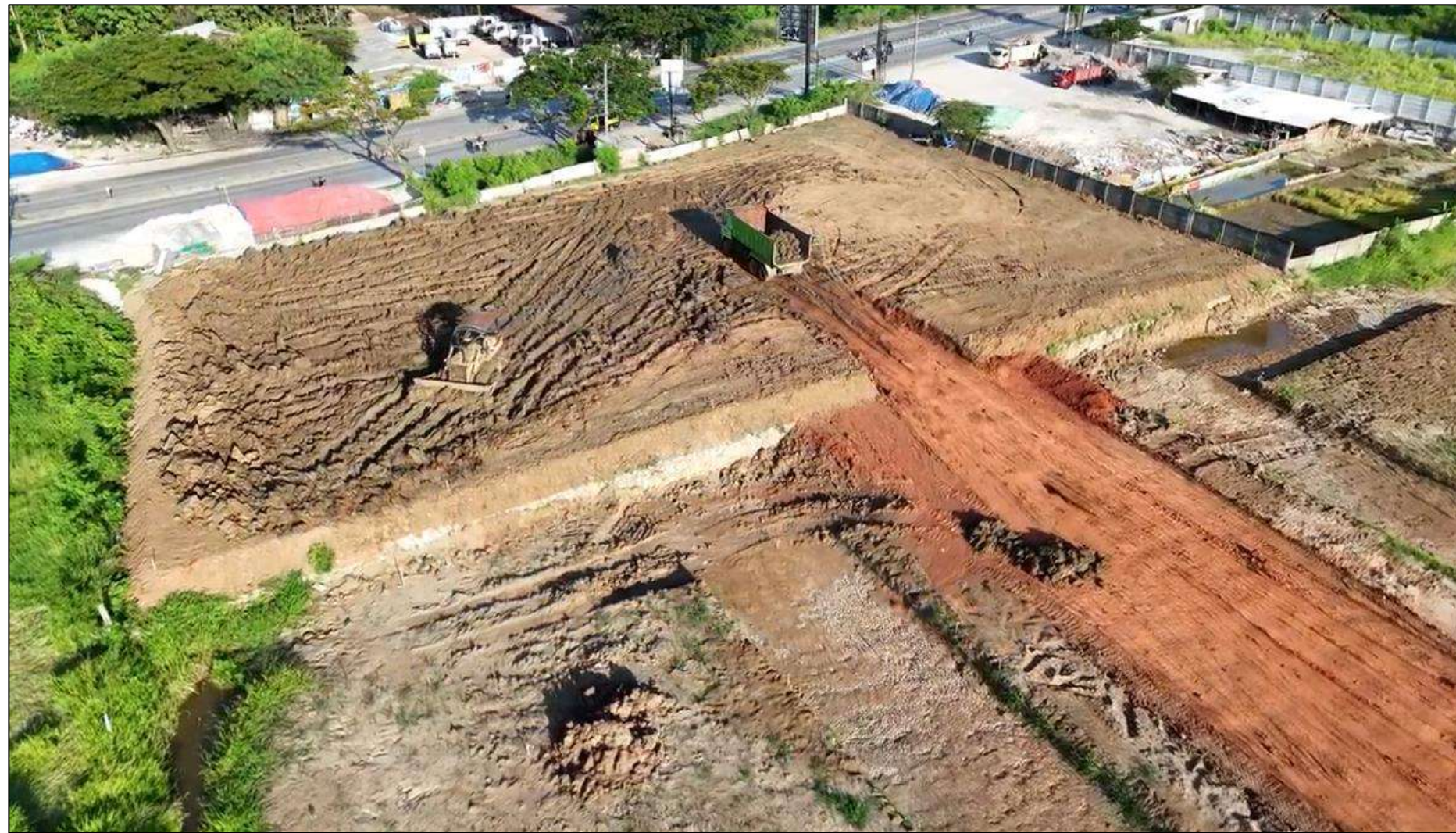
Land Clearing and Earth Filling Works for Commercial Lots
