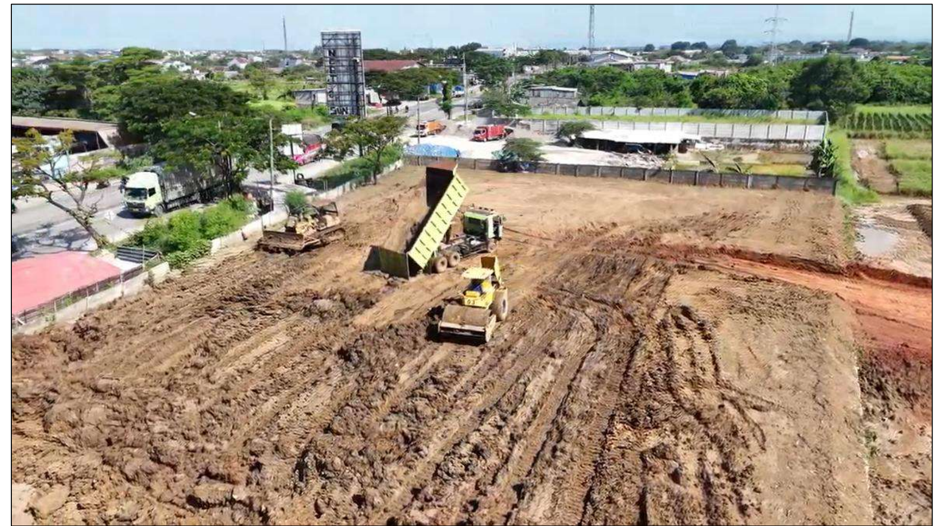
Residential Lot Formation and Road Construction Works (Eastwood Cluster)
